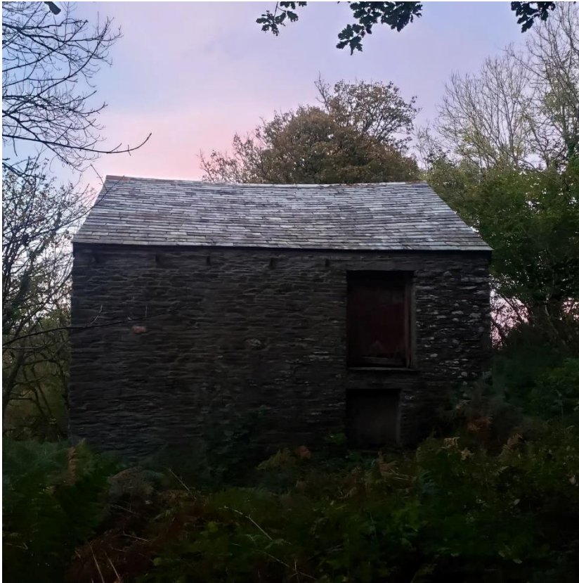
Figure 2: The Barn Behind Minster Church, site of the Boscastle Workings. Photograph by Jeff Howard.
